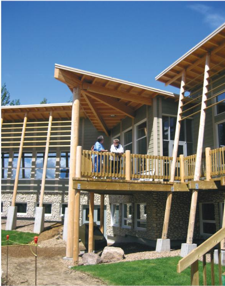
The environmentally friendly new Boreal Centre for Bird Conservation in Lesser Slave Lake Provincial Park.
