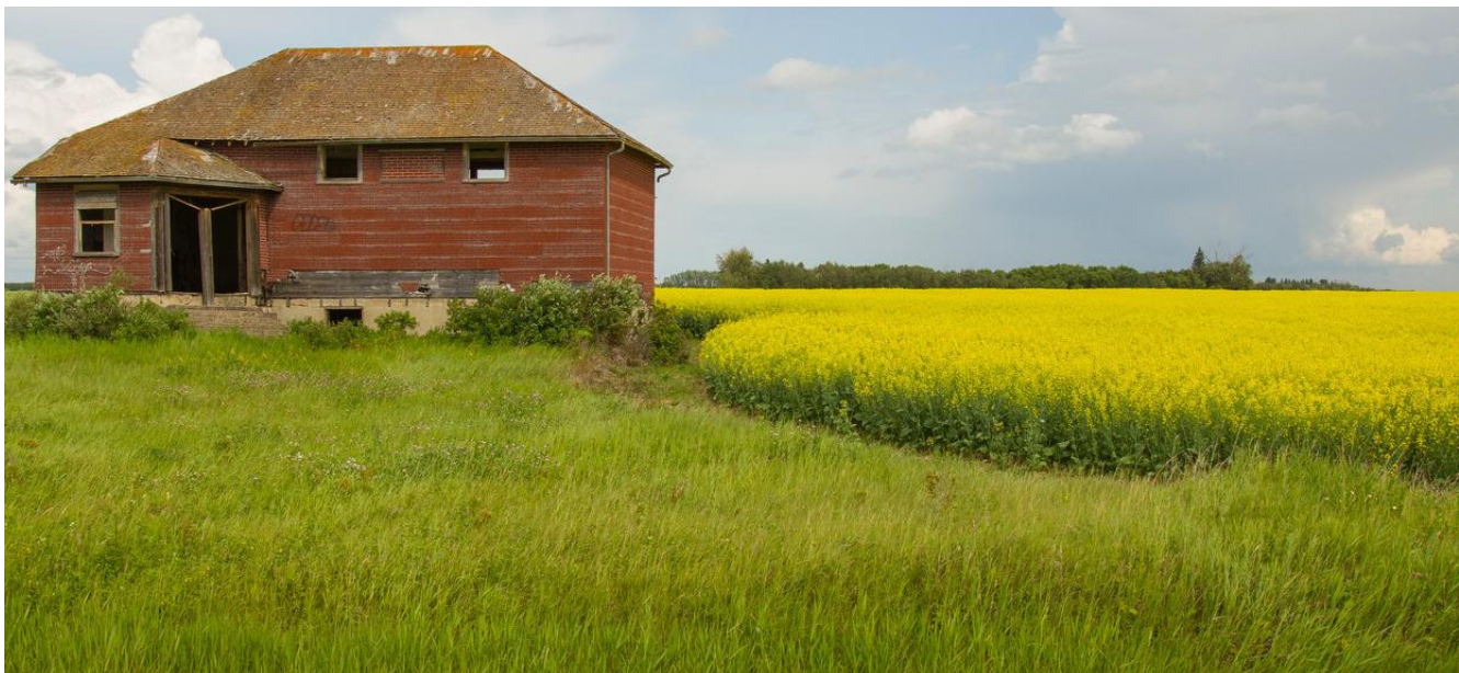
THE ALBERTA PRAIRIES, PHOTO CREDIT: MARTIN PRENTICE
